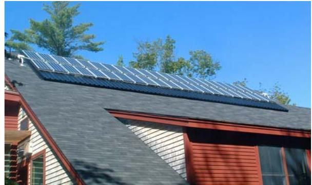
**Figure 2: PV/T air collector – SolarRoof from Conservall Engineering Inc. mounted on Chewonki Center for Environmental Education, Wiscasset, Maine, USA.**
